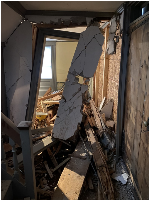
Damage to the Lindsay Road hall of the Emerson-Wilcox House as a result of a 2021 Memorial Day weekend automobile accident.
